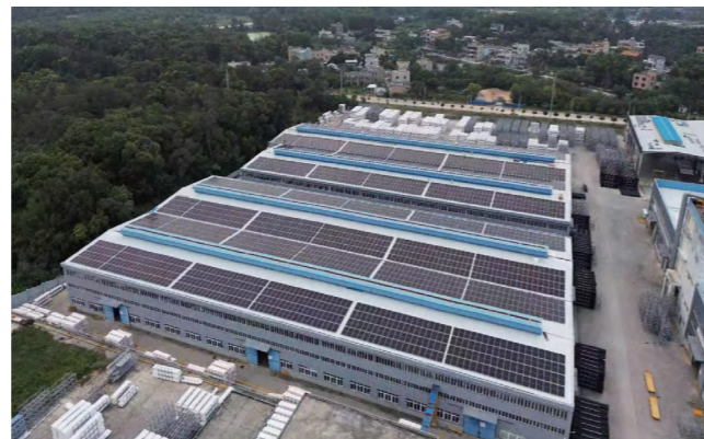
Dingan Roof Solar Power Station
