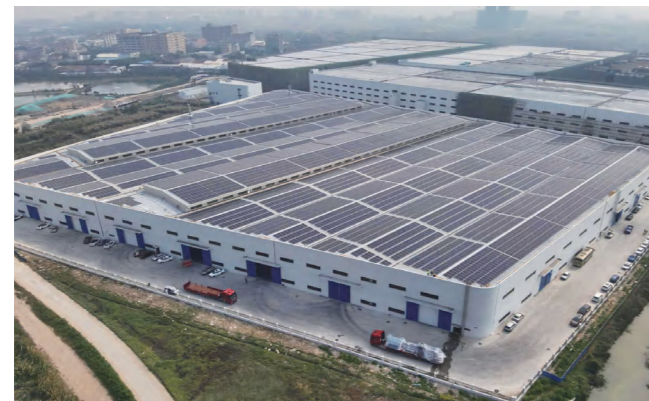
Foshan Haitian Roof Solar Power Station
