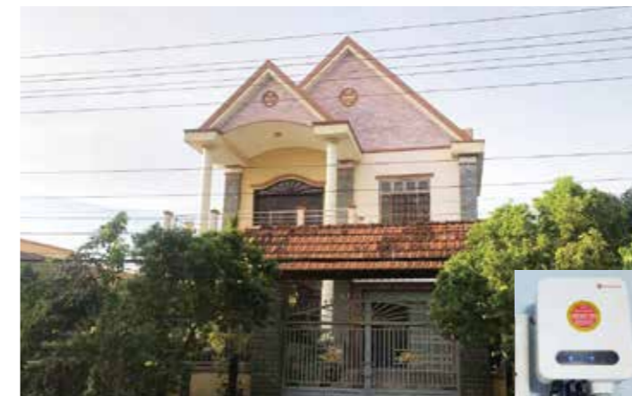
Residential PV Project in Vietnam
