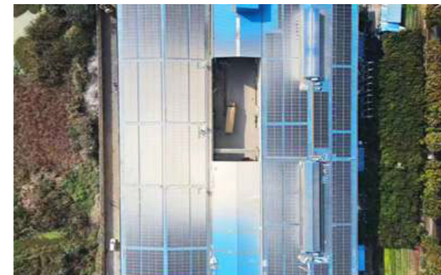
Tianfeng Rooftop Solar Power Station
